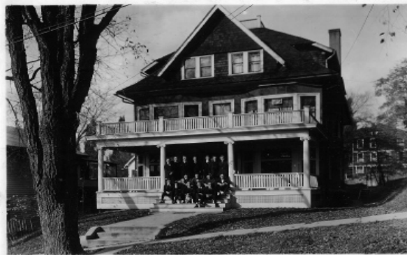
Figure 4: 614 E. Buffalo St.
