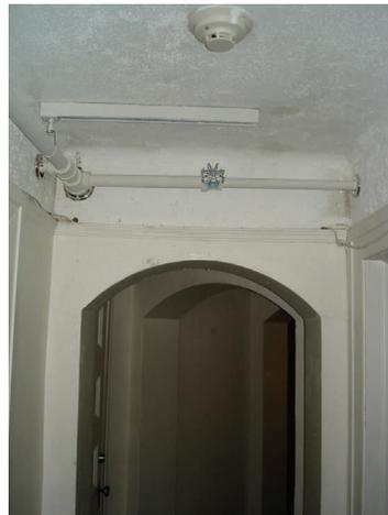
*Newly installed pipes running along the hallways on the second floor.*
